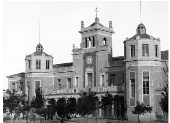
The current garden of the Music, in Elda, acted as war hospital for the International Brigades. Below, the war hospital of the Socorro Rojo Internacional in Monovar.
